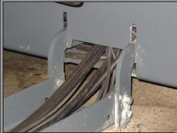
Capture bolts for the bracket are on the back side of the rear leg.
