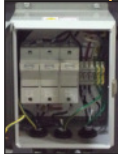
Power junction box with auto-transformer installed in the bandsaw (208V & 575V) Idler Side of the Machine
